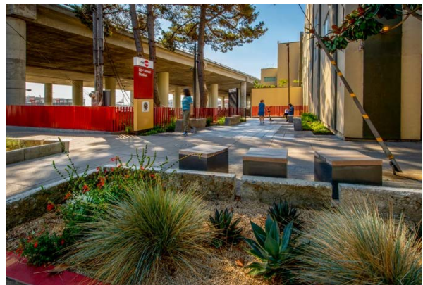
22 nd St Caltrain Station, 22 nd St at Iowa
